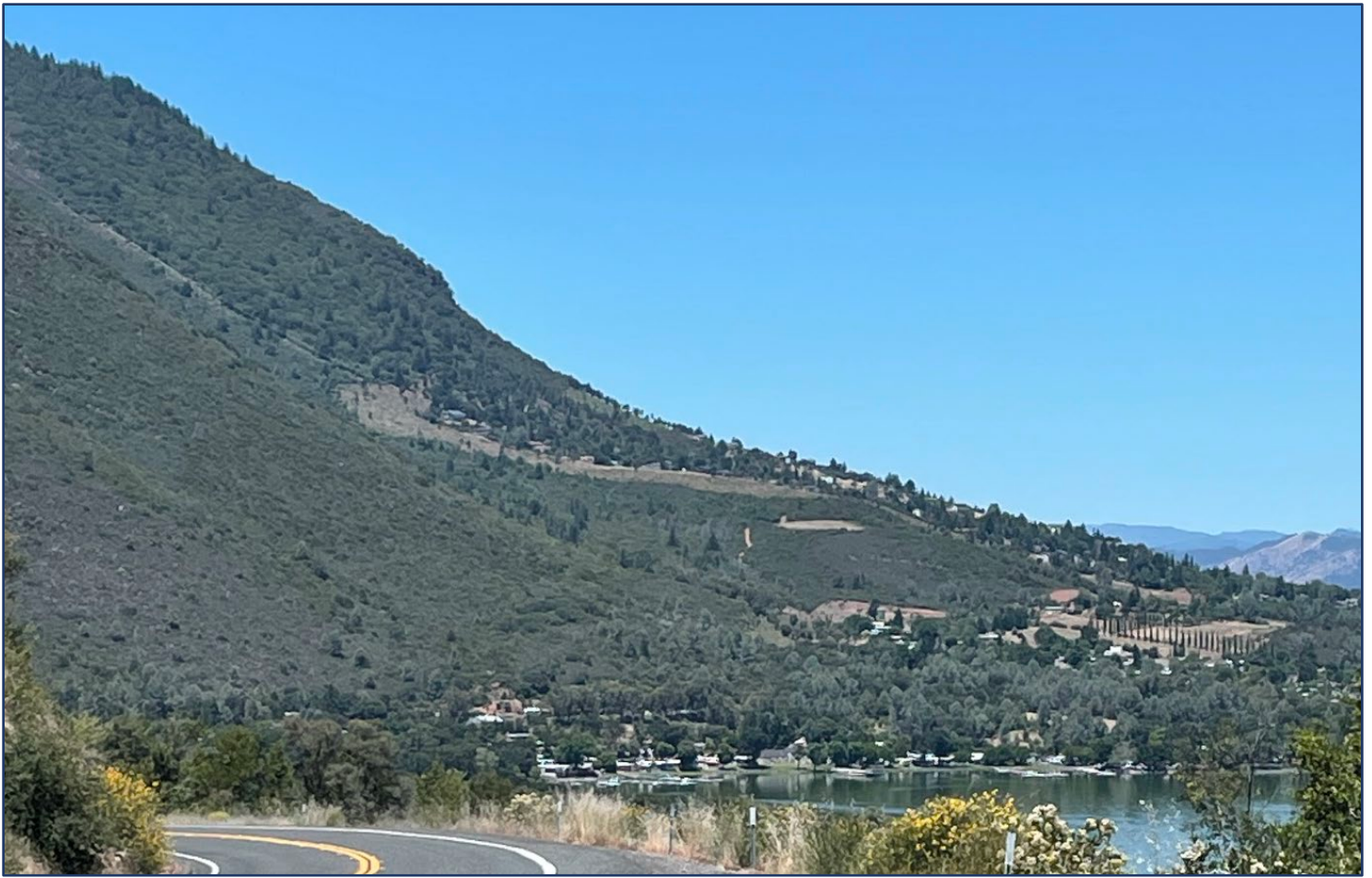
The Riviera West firebreak (center of picture) is visible as a lighter-green crescent between the residential area and undeveloped woodland.
