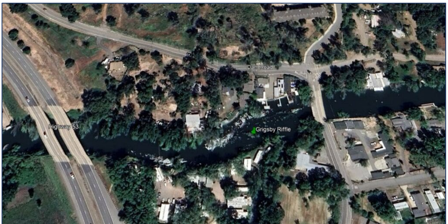
Seen near the center of this picture (YCFWCD website), the Grigsby Riffle is rock formation located in a narrow spot in Cache Creek. At left is the Route 53 bridge over Cache Creek.
